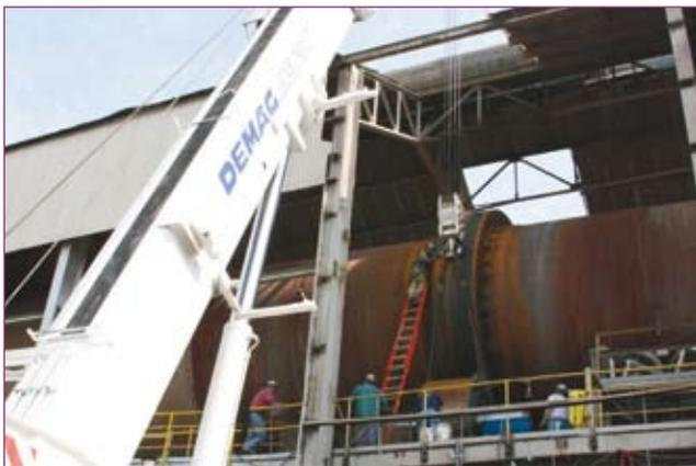
Hours after this support roller broke and shut down the kiln, EuroGear USA quickly analysed the situation and worked closely with the client to set up an emergency programme to get the kiln back up and running as soon as possible. The kiln was running 3 weeks later, versus the proposed 38 weeks by the OEM.
